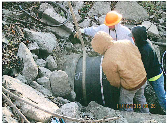
Installation of a 36" in-line check valve.
