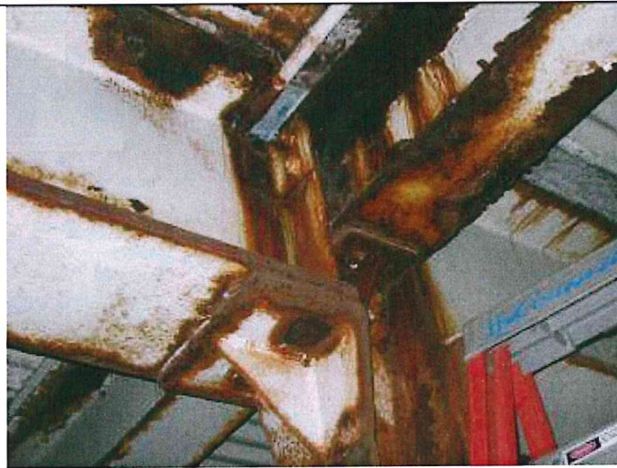
Photo 2: Deterioration and heavy rusting at structural steel joint in Parking Garage C.
