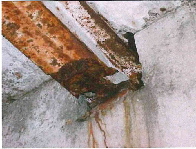
Photo 1: Beam end damage found during December 2014 inspection of Parking Garage C.
