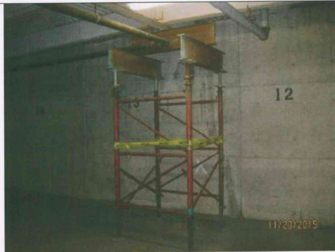
Photo 5: Shoring currently in place to support a corroded beam in Parking Garage C.
