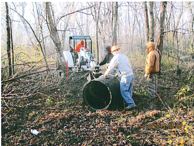
Preparing 36" in-line check valve for installation.
