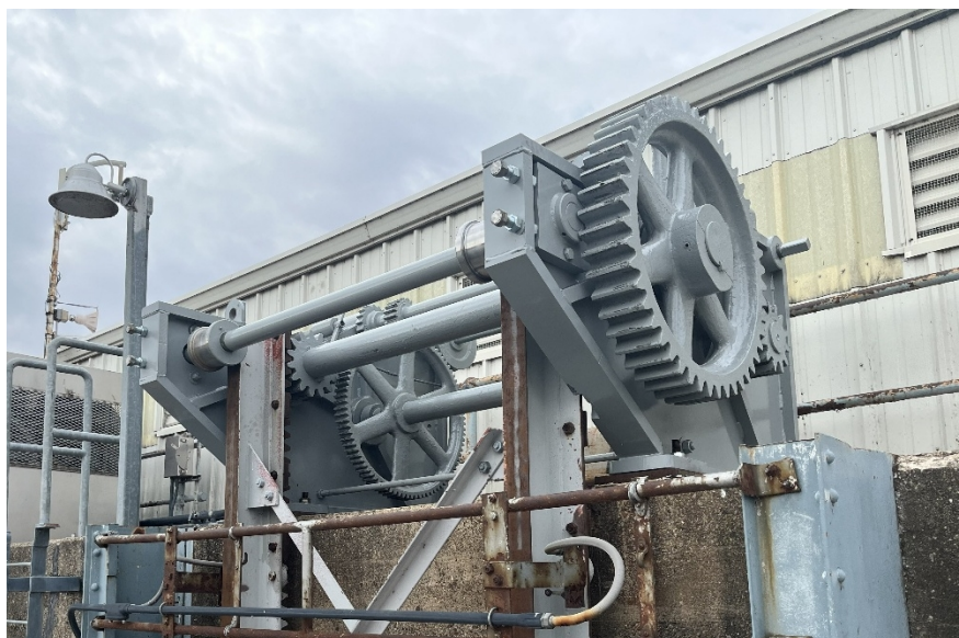
Figure 2 North Sluice Gate Machinery after Repairs; repairs to South will be similar
