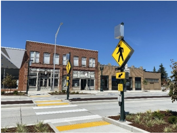
Pedestrian Crossing with Refuge, Rapid Rectangular Reflective Flashing Beacons, and Mid-Block Curb Extension
