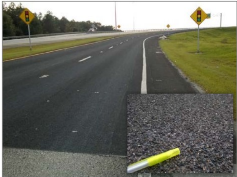
High Friction Surface Treatment in Florida
