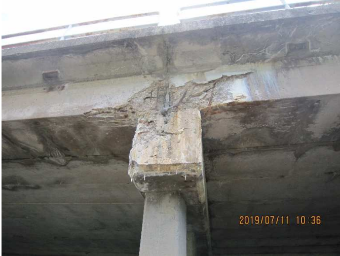
Photo 7: South end of the East Pier cap is spalling. Beams above the cap have spalled and exposed the reinforcement.
