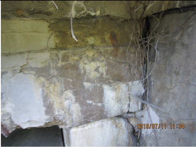
Photo 8: End of Beam 11 above the East Abutment.
