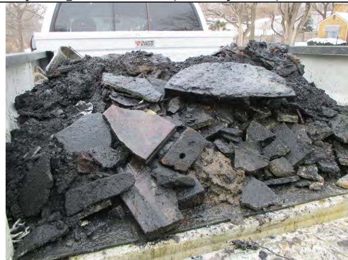
Material that is being pulled by hand from the sewer during the cleaning process. (Courtesy BGM)
