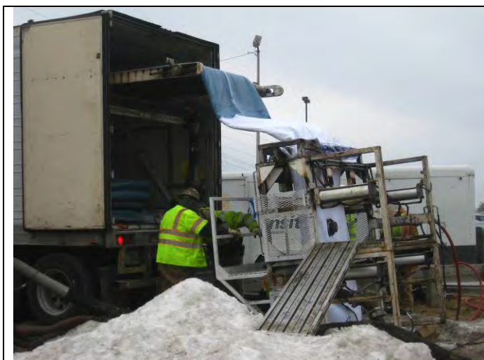
Liner being fed into the sewer near St. Mary's Hospital. Note the white section that does not contain the blue resin. This is so that it will not adhere to the manhole before it gets to the sewer.
