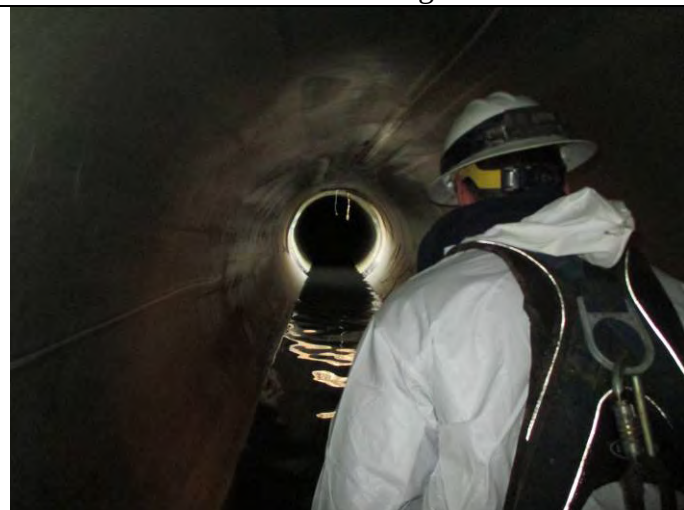
Inspecting the new liner. (Courtesy BGM)
