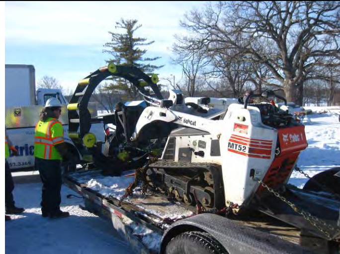
The spiral winding unit is mounted to a Bobcat tractor that will back down the sewer as the liner is wound into place.
