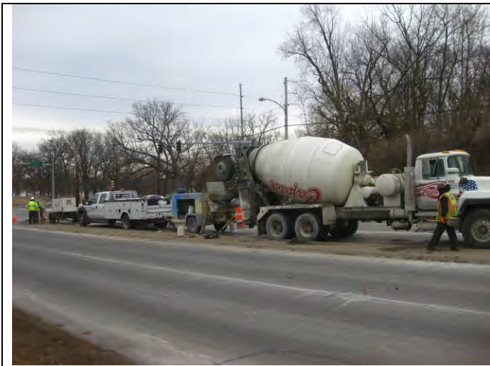
Concrete grout is pumped into the sewer to form a smooth floor as the base for the spiral liner.
