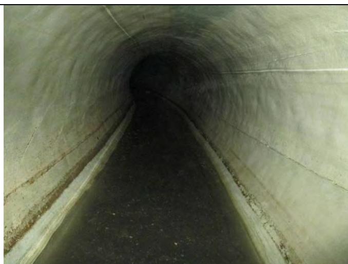
Newly lined 84" sewer at Lake Shore Drive and MLK. (Courtesy BGM)
