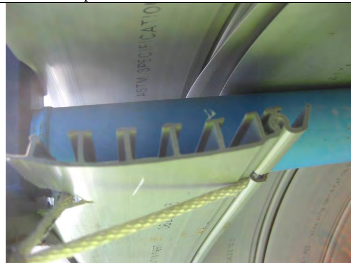
Close-up of the cross section of the PVC liner panel. This is for your information.
