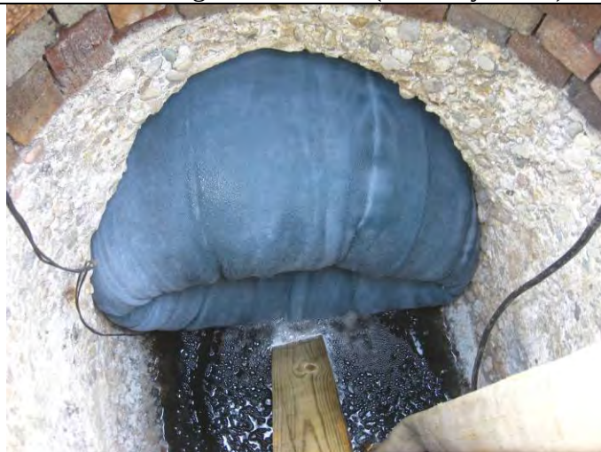
Cured-in-place liner inflating into a manhole.
