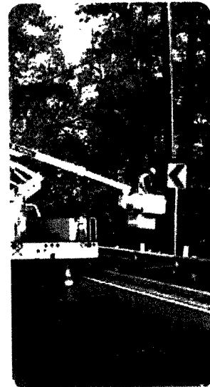
City Foot Traffic Street Electric & existing pole
