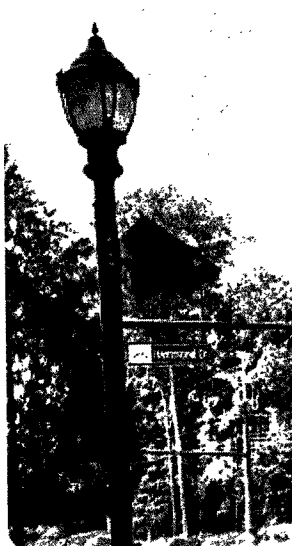
City intersection Solar & existing pole
