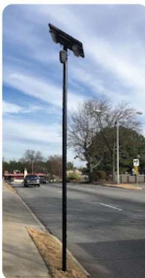
Entrance to Hotel Solar & Flock 14 foot pole
