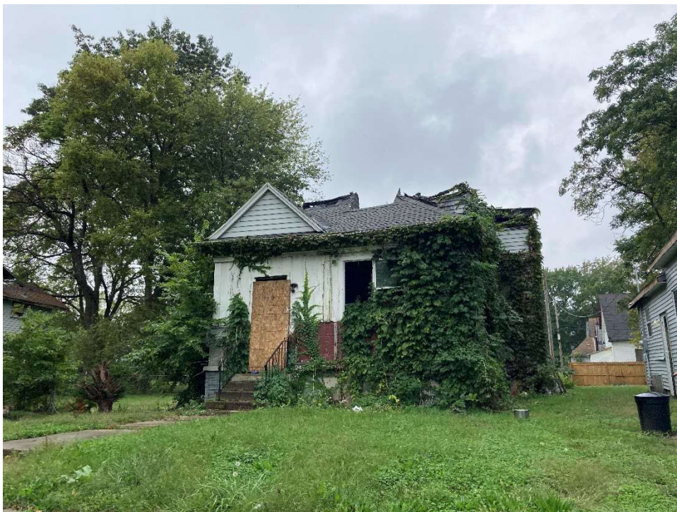
Figure 4-8: Demolitions are still needed in some areas
