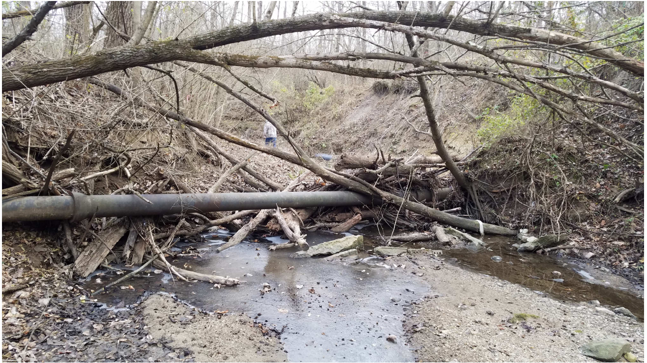
Photo 1: faces upstream shows two pipe joints exposed with no support
