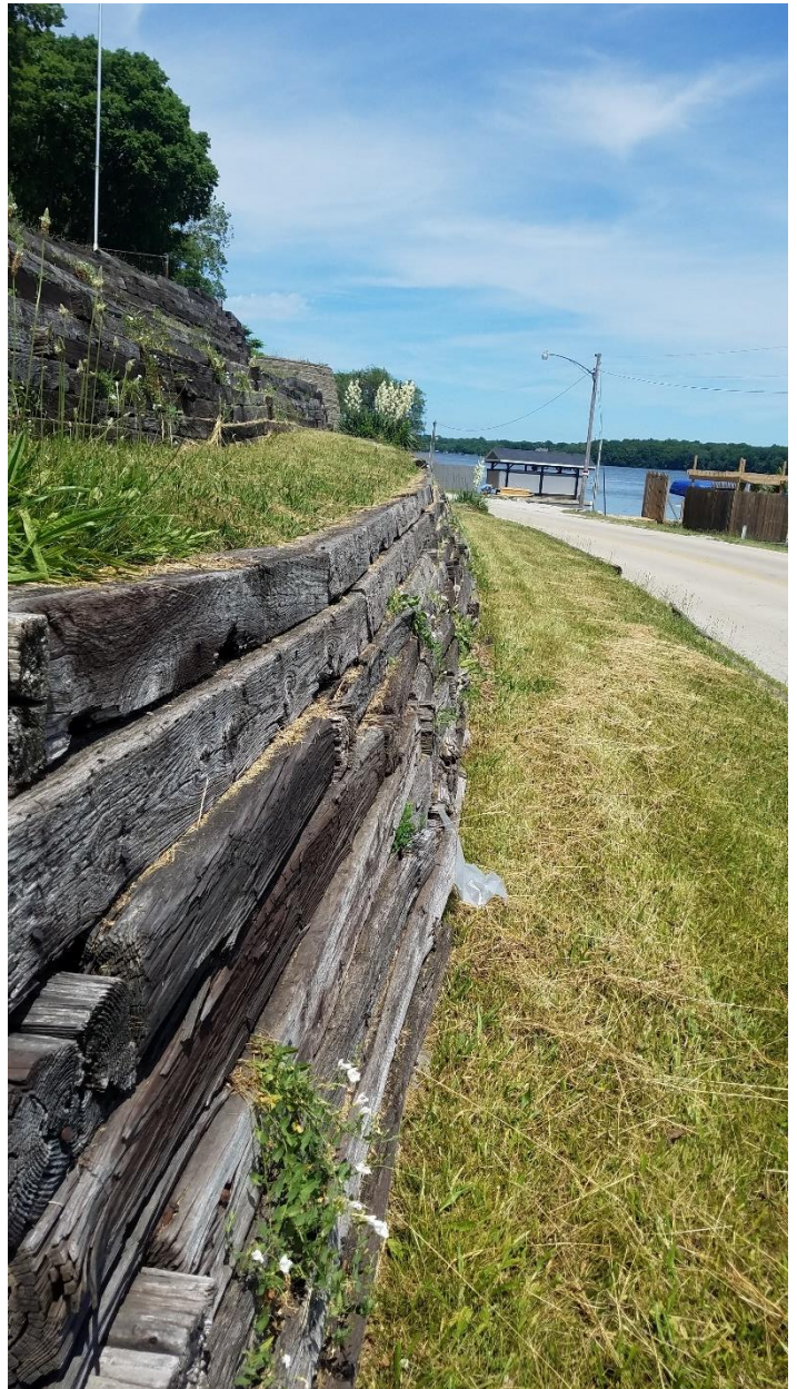
Photo 3 and 4: Shows the condition of the existing wall and stairs. The condition of the railroad ties is poor with many railroad ties rotted out.
