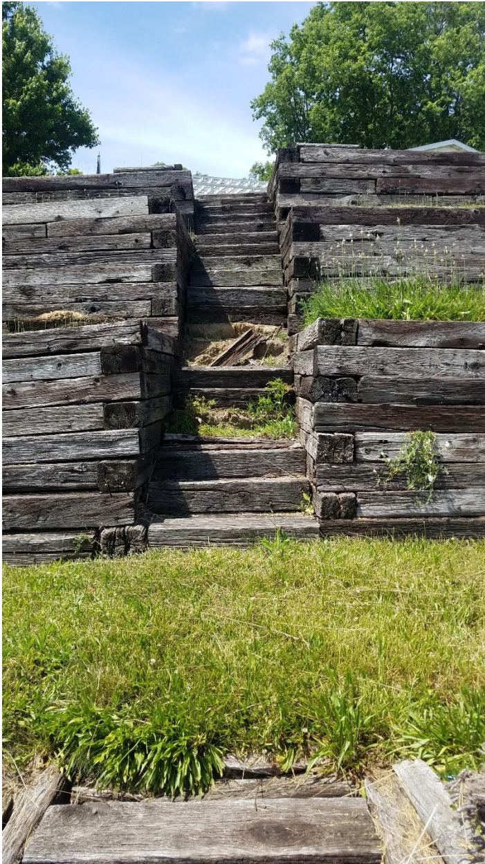
Photo 3 and 4: Shows the condition of the existing wall and stairs. The condition of the railroad ties is poor with many railroad ties rotted out.
