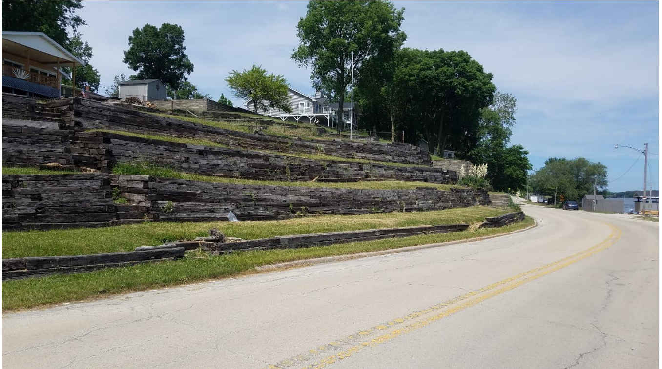
Photo 1: Side view of the wall looking northeast. The block wall built in 2000 is located at the far-right side of the wall
