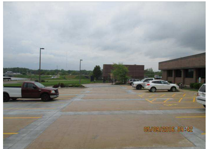
South Water Treatment Plant parking lot completed
