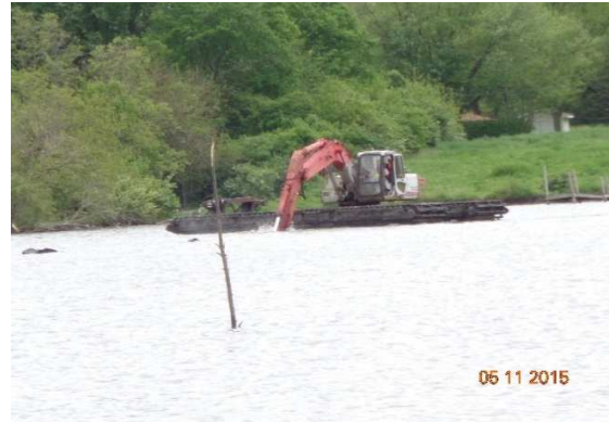
Swamp excavator at work digging up stumps in Big Creek Basin.
