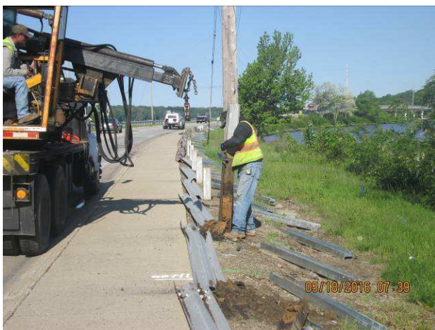
Removing the old guardrail.
