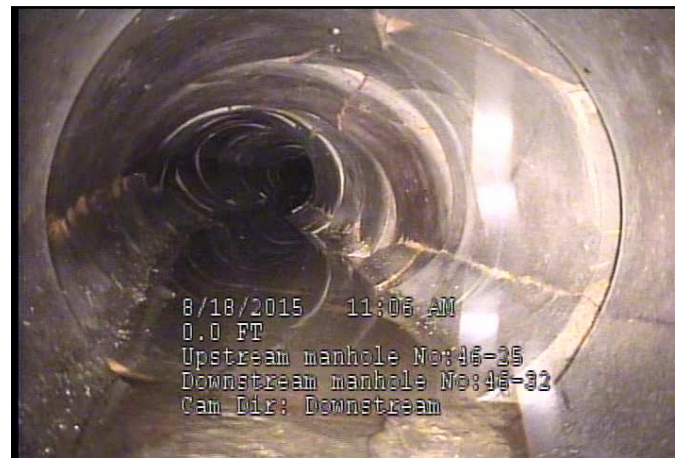
4. Section of pipe showing a near collapse condition. Fairview Park.
