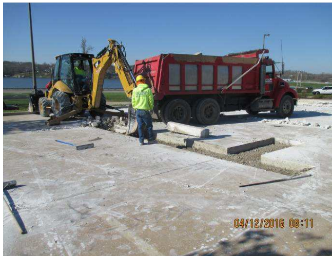
South Water Treatment Plant parking lot under repair
