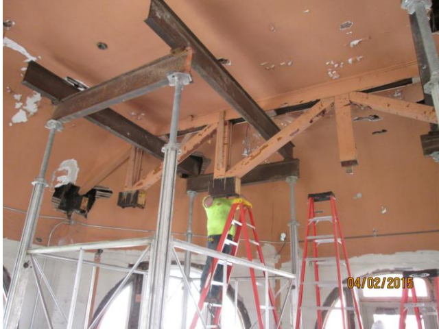
Removing Bottom Chord
