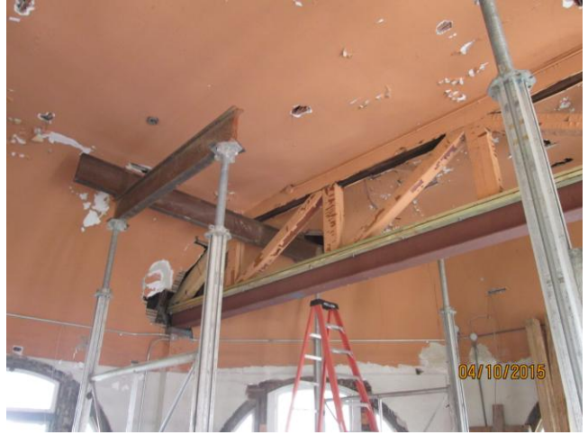
New Bottom Chord in Place
