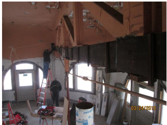
Preparing To Remove Bottom Chord
