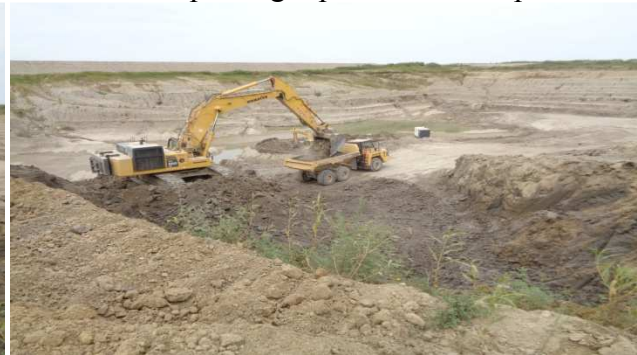
Excavator with 8 yard bucket at sedimentation basin. It takes 3 scoops to fill a 40 ton dump truck.
