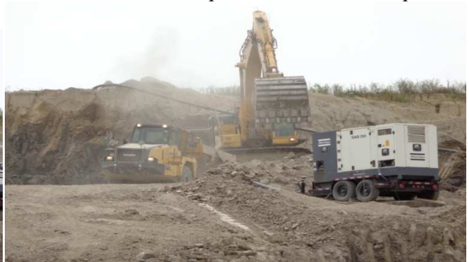
Excavator with 8 yard bucket at sedimentation basin. It takes 3 scoops to fill a 40 ton dump truck.
