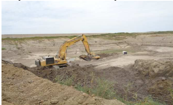
Excavator with 8 yard bucket at sedimentation basin. It takes 3 scoops to fill a 40 ton dump truck.
