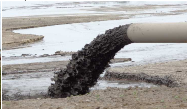
Discharge of lake sediment and lake water at the end of the dredge pipeline with a close up view.
