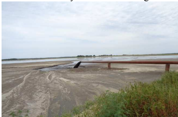
Discharge of lake sediment and lake water at the end of the dredge pipeline with a close up view.
