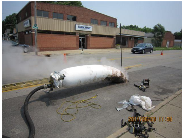
Heat curing of felt tube liner.
