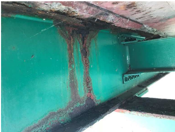
Pack rust on south beam near cross beam. Some rusting on cross beam
