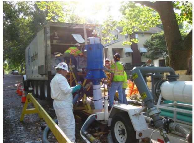
Inserting the liner into the pipe.
