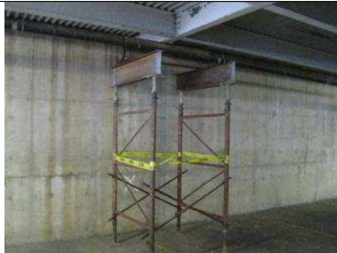
Photo 4: Shoring currently in place to support a corroded beam in Parking Garage C.
