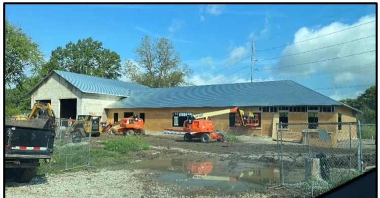
New Station 7 construction
