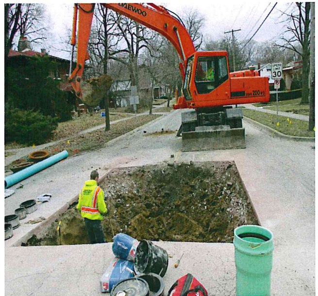
Replacing a failed manhole at the intersection of W. Main St and Woodlawn Ave.
