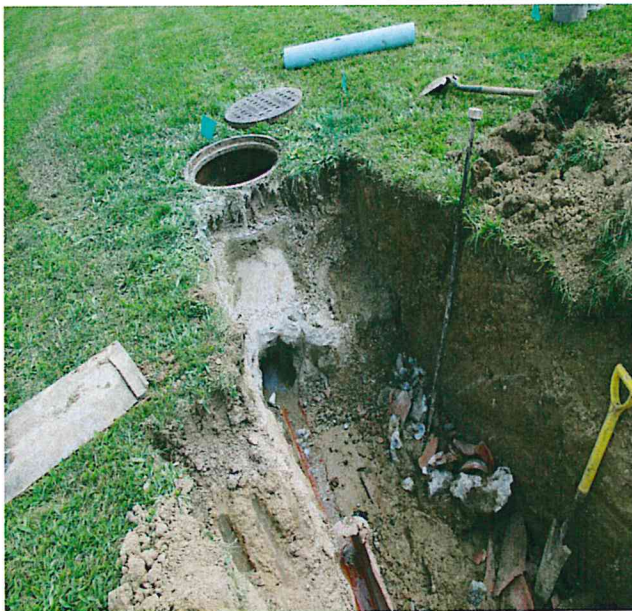
Repairing a failed section of sanitary sewer near W. Terrace Dr in South Shores.
