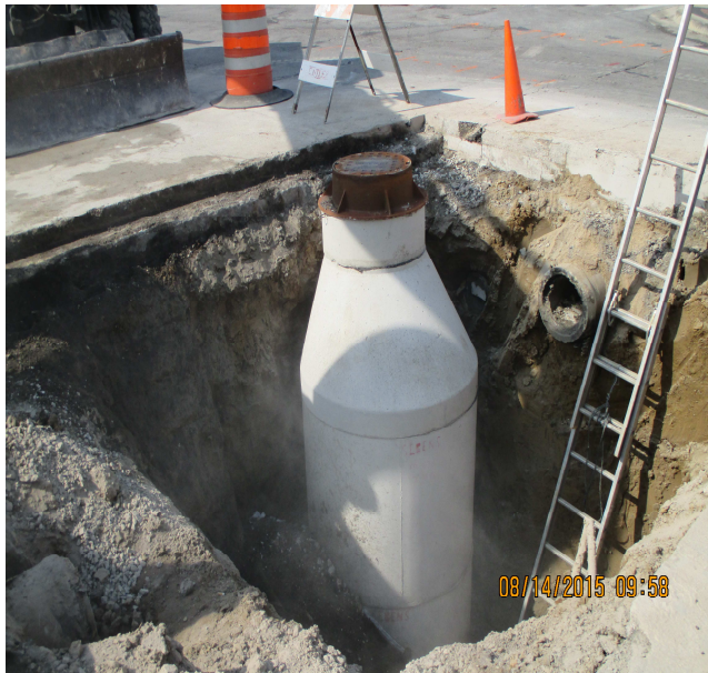
New manhole installed at the intersection of E North St and N Franklin St
