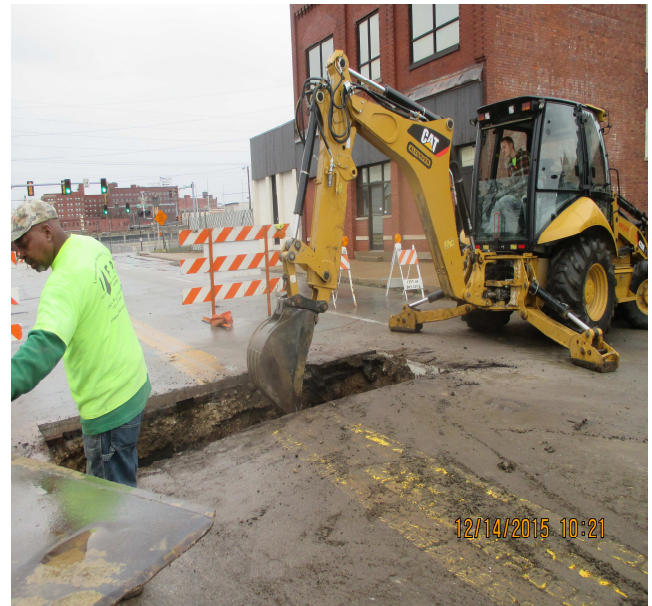
Sanitary sewer repair at E Wood St
