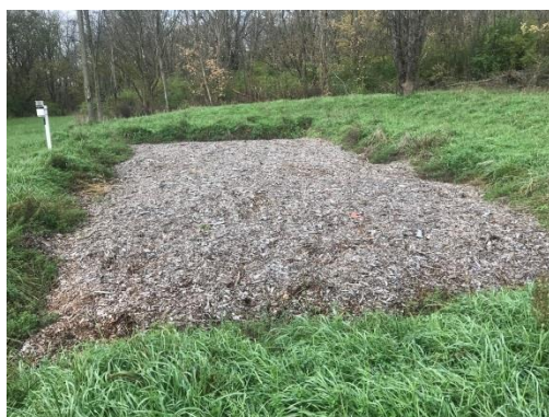
RCPP denitrifying woodchip bioreactor north of Argenta in Friends Creek subwatershed.
